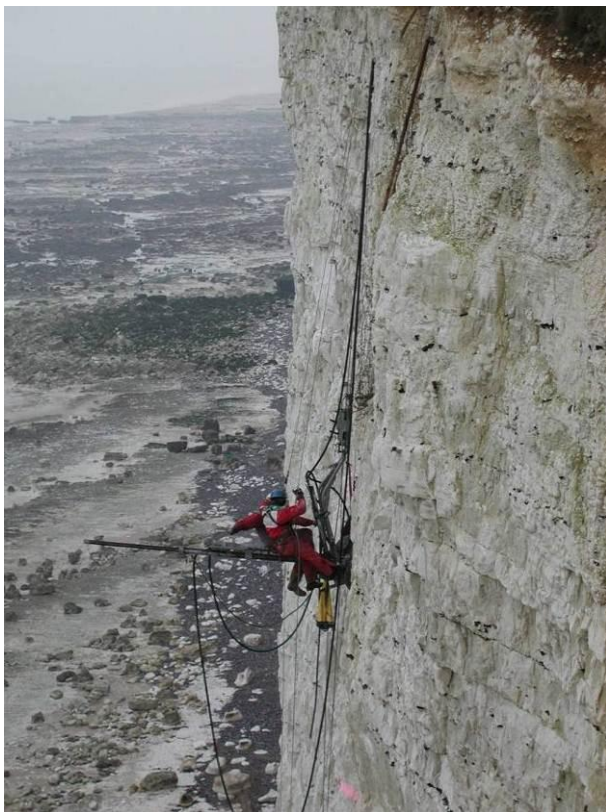
Figure 32. Drilling horizontal boreholes at Mesnil-Val for the PROTECT Programme
