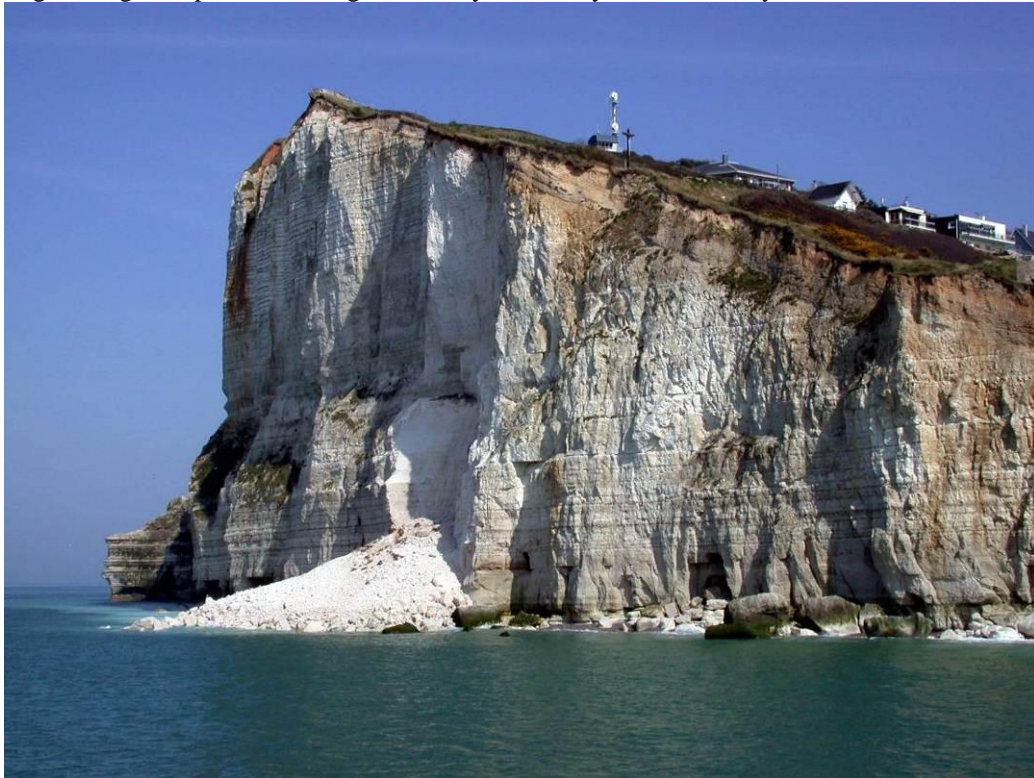
Figure 24. Cliffs at Fécamp on the north side of the Fécamp Fault
