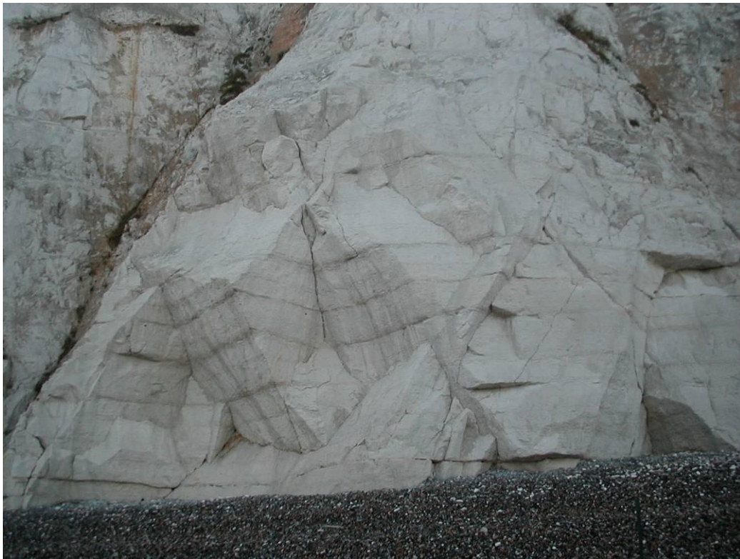
Figure 29. Inclined conjugate fractures in the Holywell Chalk at St Martin Plage
